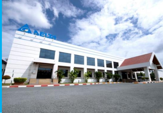
Bangpoo Plant – Plant 1
