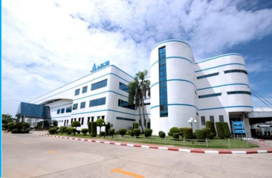
Bangpoo Plant 5 (HQ)
