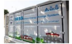
2MW/1MWh Energy Storage System for Xia Xing Power Station on Kinmen Island
