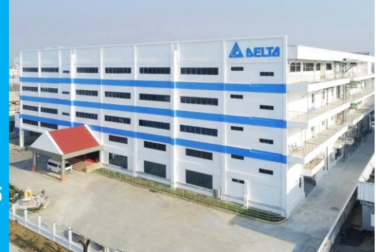
Bangpoo Plant – Plant 3
