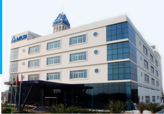
Gurgaon Plant (Head Office)
