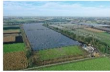
1,500 PV inverters for the largest ground-mounted solar park in Southern Germany.
