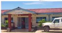
Renewable energy solutions featuring subsidiary Eltek's Rectifier for 104 Hospitals in Zimbabwe under the UNDP's program
