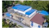
Modular containerized data center solution for a submarine cable landing station in Myanmar
