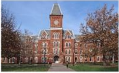
Building management solutions provided by subsidiary Delta Controls for more than 180 buildings at a university in the eastern U.S.
