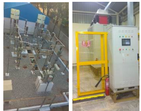
PQR Lab, left side-outdoor yard, Right side indoor lab
