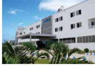
Rudrapur Plant (Green Building)
