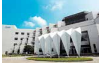
Tainan Plant (Diamond-rated Green Building)
