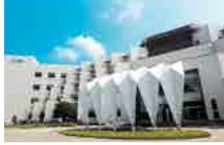
Tainan Plant (Diamond-rated Green Building)
