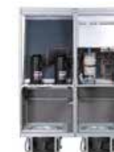
Fans under raised floor provide same air flow with 20% less power consumption
