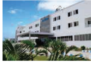
Rudrapur Plant (Green Building)
