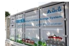
2MW/1MWh Energy Storage System for Xia Xing Power Station on Kinmen Island
