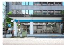
EV Charging Station that is capable of assisting disaster response for the city of Yokohama
