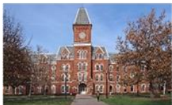
Building management solutions provided by subsidiary Delta Controls for more than 180 buildings at a university in the eastern U.S.
