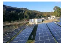
4.6 MW distributed solar power system with energy storage system in Ako, Japan
