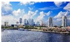
Building control system for a luxury hotel in Tampa Bay
