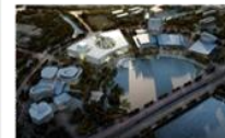
Building management solution from subsidiary LOYTEC for Yangzhou Canal Grand Theater in China
