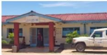
Renewable energy solutions featuring subsidiary Eltek's Rectifier for 104 Hospitals in Zimbabwe under the UNDP's program
