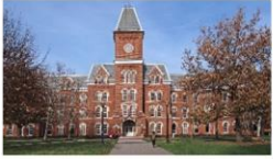
Building management solutions provided by subsidiary Delta Controls for more than 180 buildings at a university in the eastern U.S.
