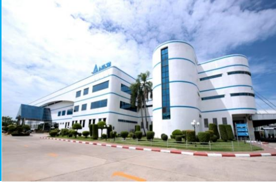
Bangpoo Plant 5 (HQ)
