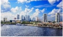
Building control system for a luxury hotel in Tampa Bay
