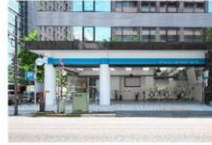
EV Charging Station that is capable of assisting disaster response for the city of Yokohama
