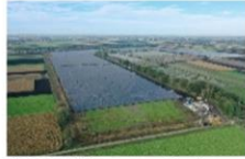
1,500 PV inverters for the largest ground-mounted solar park in Southern Germany.
