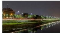
Smart streetlight total solution including 21,000 LED streetlights for smart city project in Jakarta
