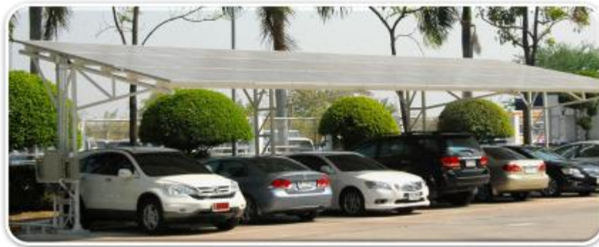
Solar panel installed on the roof of the parking lot to generate 11 kilowatts of electricity to use in the Company's lobby.
