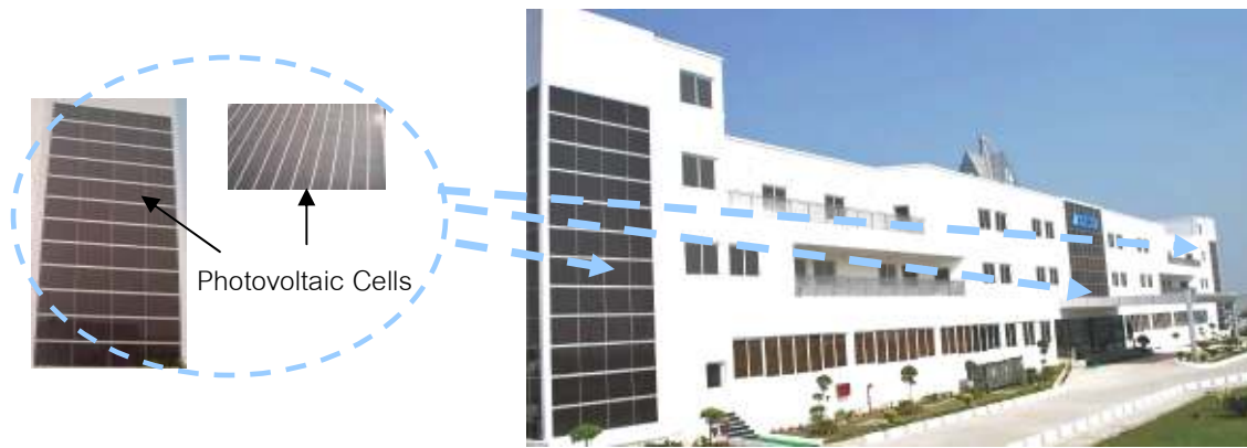
Solar panel installed on the outside wall of the Rudrapur plant (India) for power generation
